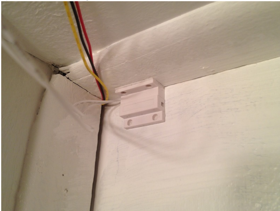
Magnetic door switch contacts have sticky foam, or screws for a more permanent install.
