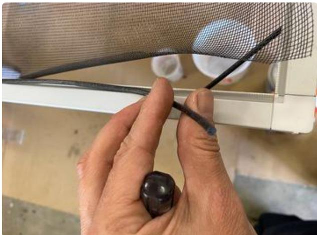
Use a flat head screwdriver to pry out the foam rubber spline in the frame's groove. Pull it out completely and set it aside.
